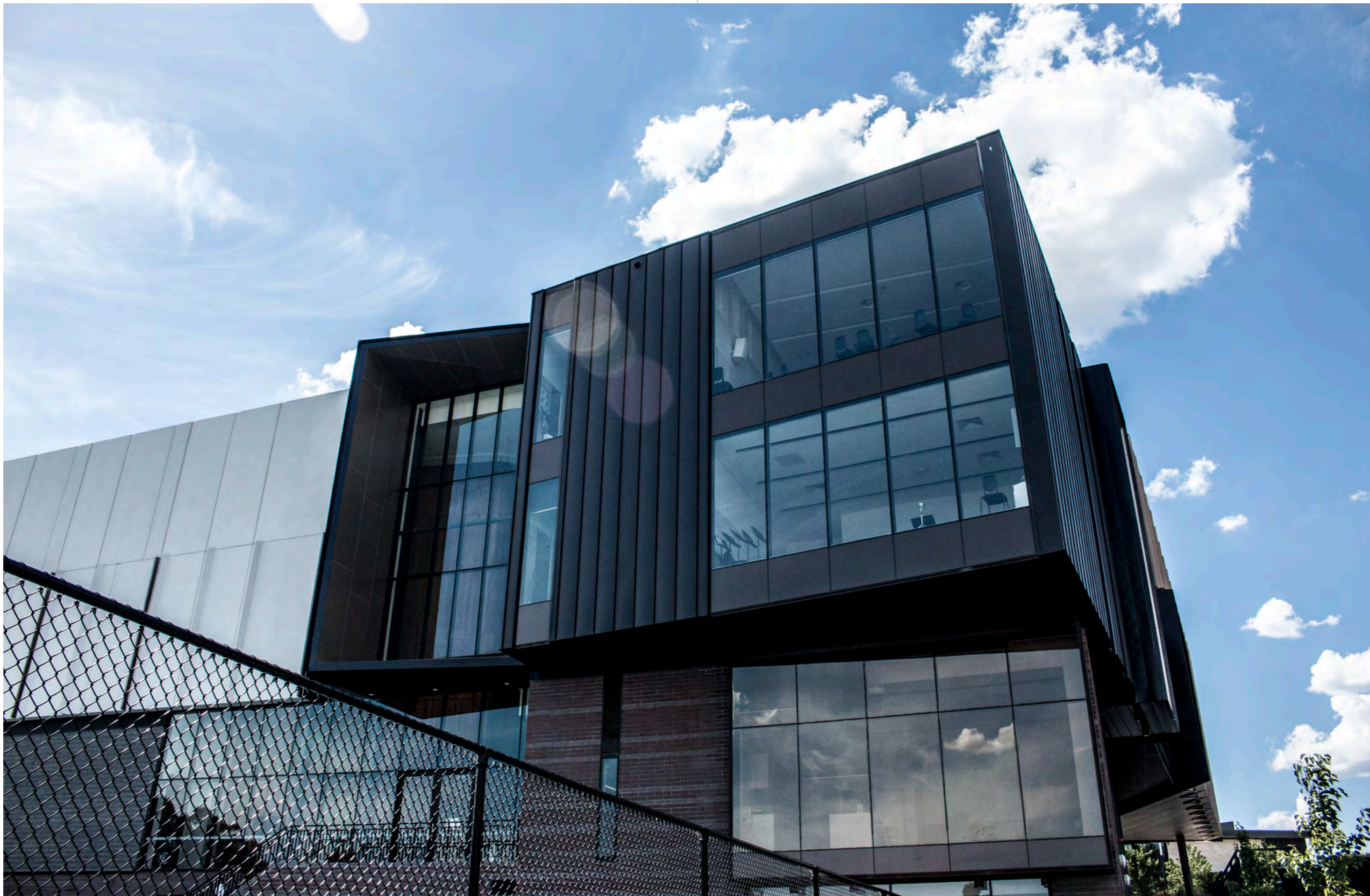
PRESBYTERIAN LADIES COLLEGE, PERFORMING ARTS CENTRE - MELBOURNE Vestis: Black Graphite System: Interlocking and Standing Seam Architect: Cox Architects
