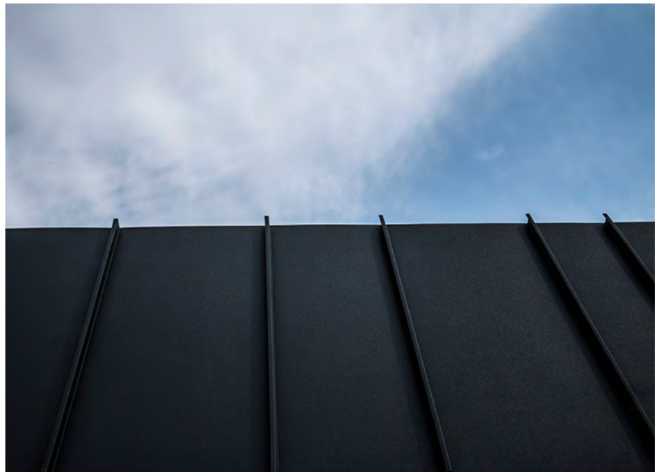
BATES STREET HOUSE - MELBOURNE Vestis: Nebula Luna and Nebula Midnight System: Standing Seam and Interlocking
